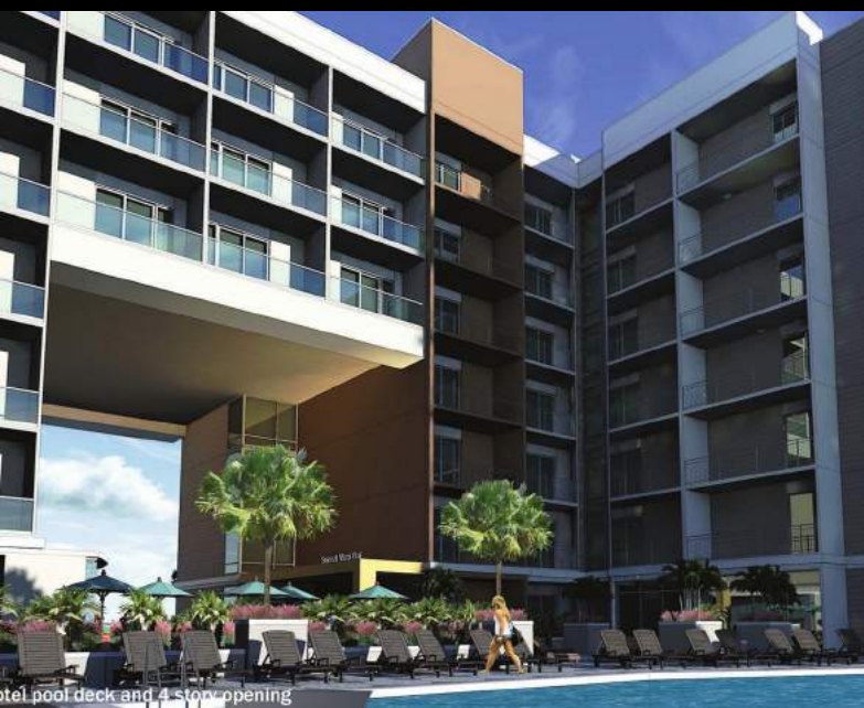
View of 5th Floor Hotel Pool Deck and 4 Story Opening
