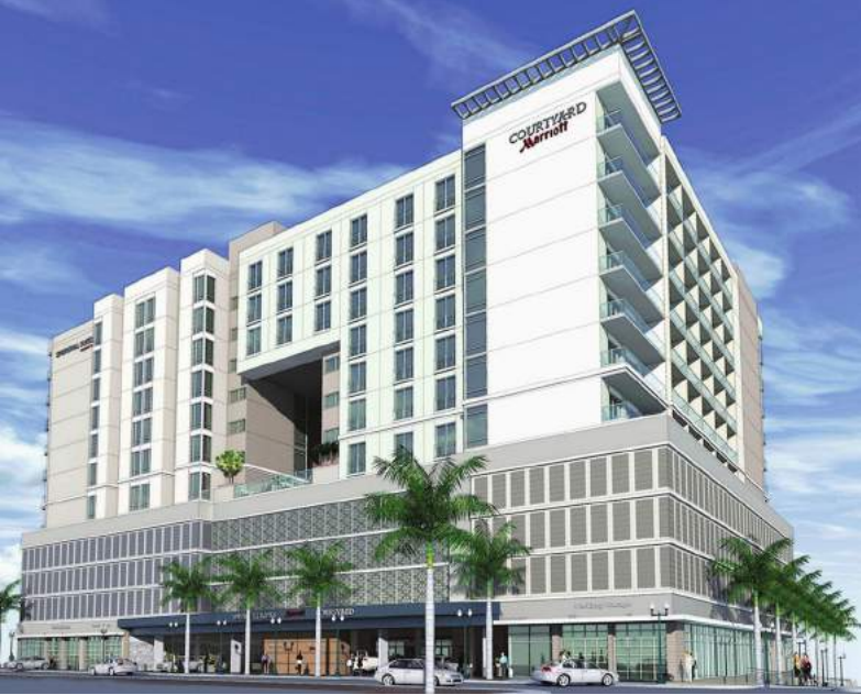
Ground Level View From SW Corner
